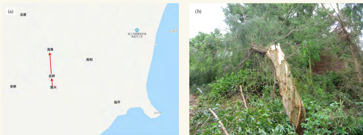
图1 龙卷移动路径(a)及受灾现场图片(b) Fig. 1 Tornado path (a) and damage picture (b)
